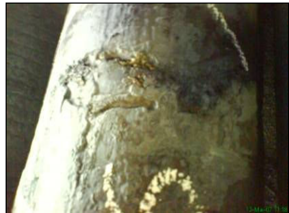
Figure 14. Breaking the casting
